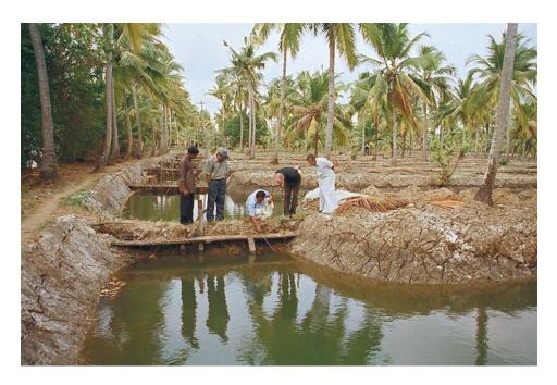
Small dams were built in water channels to make the 250-squaremeter test ponds.
