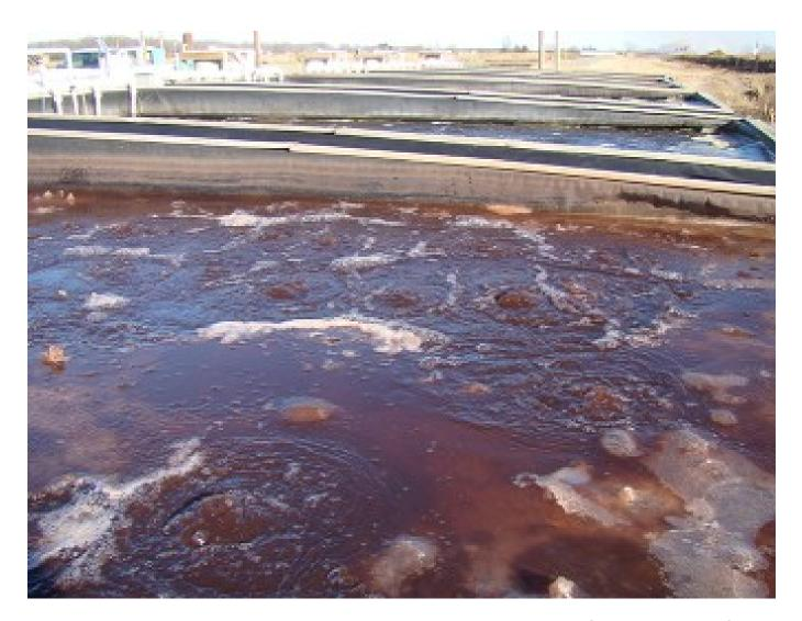
During the coldest temperatures, ice was observed covering up to a maximum of about 75 percent of the tank surfaces.
