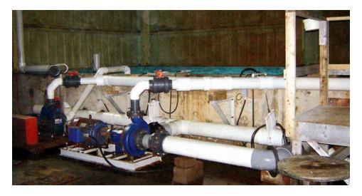
Properly configured supply pipes provide the unobstructed water flow that helps limit cavitation.
