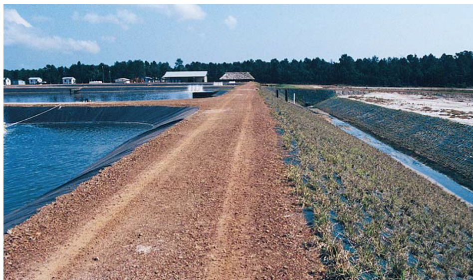
Pond levee showing plastic liner on left (wet) slope. Right (dry) slope is covered with fabric mesh and sprigged with grass to control erosion.
