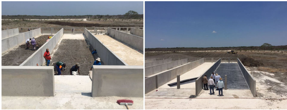
View of raceway construction for the demonstration project.
