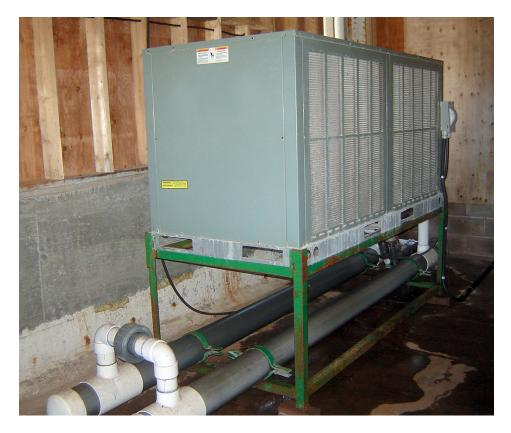
The shell-and-tube evaporators underneath this air-cooled condenser were designed specifically for the low flows and low temperatures often found in aquaculture hatcheries.
