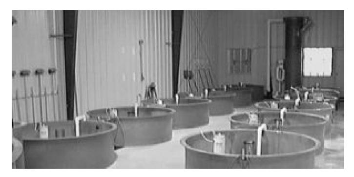
Before water enters the fry tanks, a nonpressurized packed oxygen column (behind culture tanks in this picture) adds pure oxygen to the water while driving out dissolved nitrogen.
