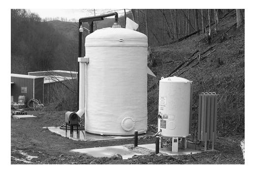
Mine water is pumped to an aeration column built into the top of a reservoir tank located above the MCRA Hatchery building where arctic char are cultured.
