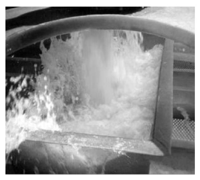
Water is broken into droplets as it flows through a counter-current forced-air cascade stripping column installed in the top portion of a water reservoir tank at the MCRA Hatchery.
