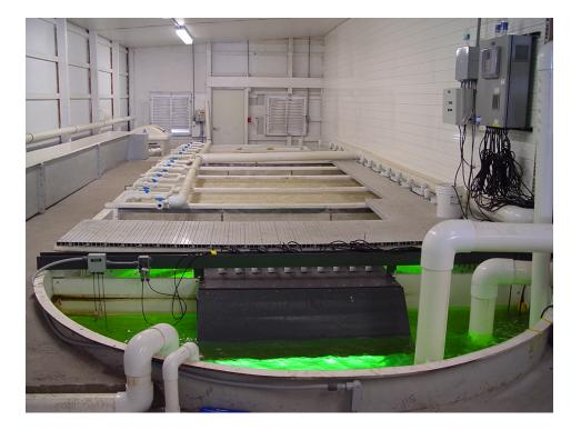
Even if a facility has a properly sized or even oversized biofilter, as in this large moving-bed biofilter with ultraviolet treatment, yet the flow between the biofilter and culture tank is too slow, the biofilter capacity will never be fully utilized, and ammonia nitrogen can build up in the culture system. Photo courtesy of Mote Marine Lab.
