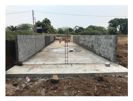
View of the demonstration in-pond raceway during construction. Note the fixed, cement floor on the pond bottom.
