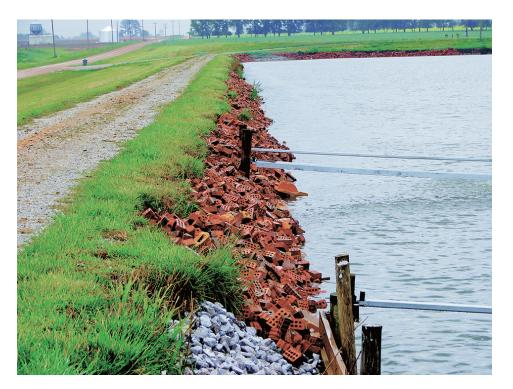
Rip-rap – even used brick – can protect levees from erosion and extend the useful life of culture ponds.
