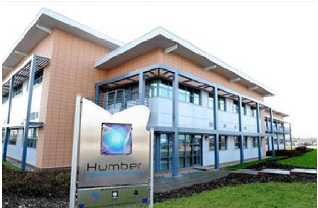
The aquaculture center will be located at the Humber Seafood Institute in Grimsby.
