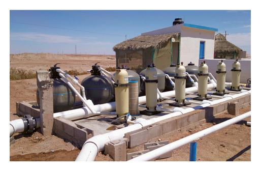
Raceways with zero water exchange employ filtration systems, aeration and other equipment to maintain a stable rearing
