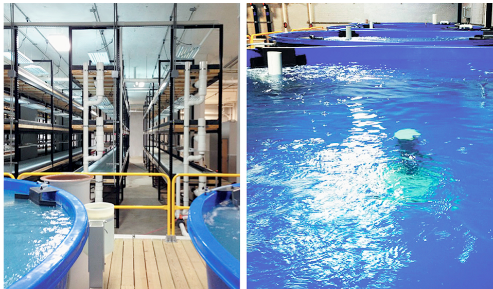
At the Hamm's Brewery project, fish culture tanks recirculate water with three-tiered racks of plant-growing trays.
