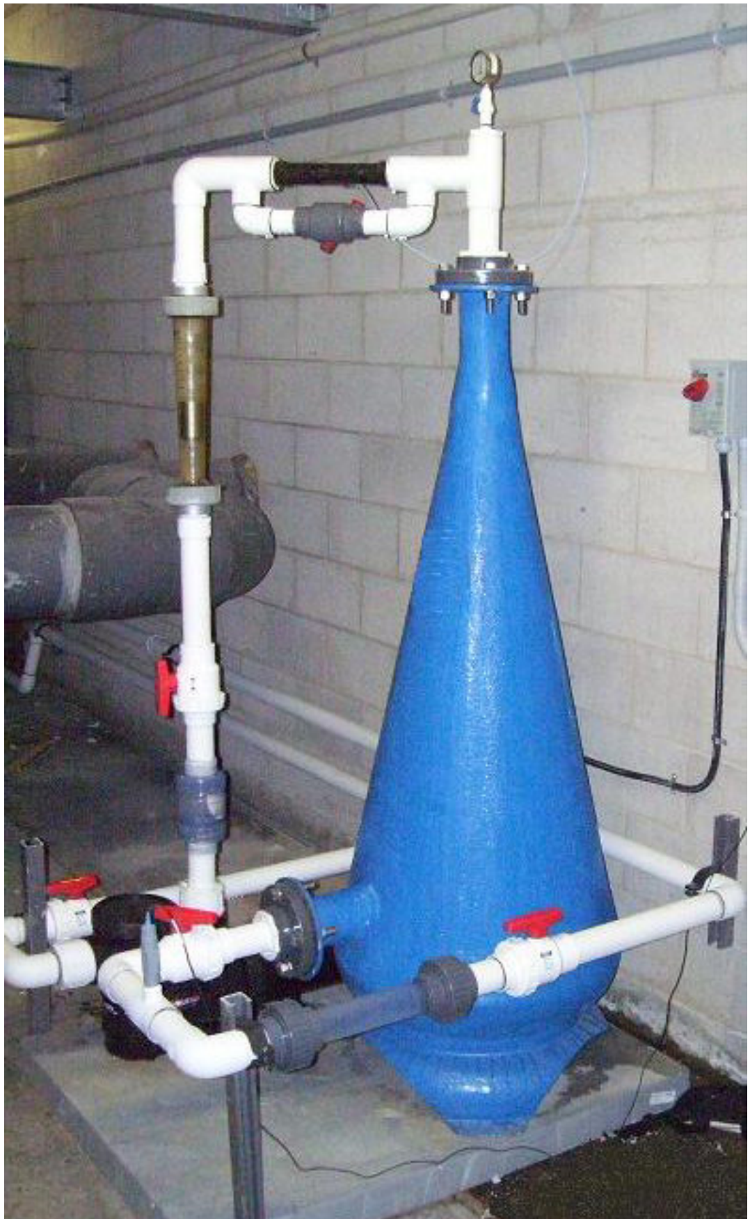
Oxygen cones are fairly easy to install and operate, and require no maintenance.
