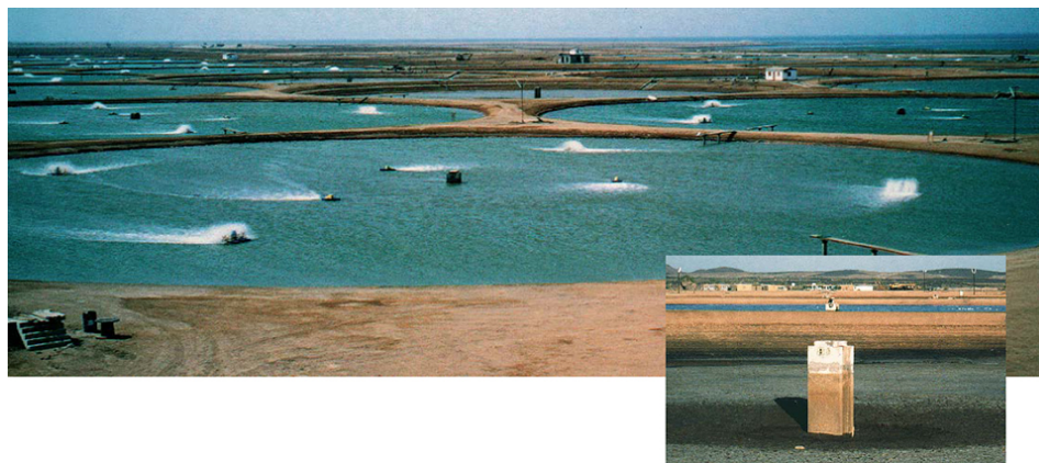
Fig. 2: This view of a production pond shows the tip of the central drainage structure and the current created by the aerators: four paddlewheels on the outer circle, and three air injectors in the center. Inset: Central drain and clean bottom with no black deposits four days after harvest.
