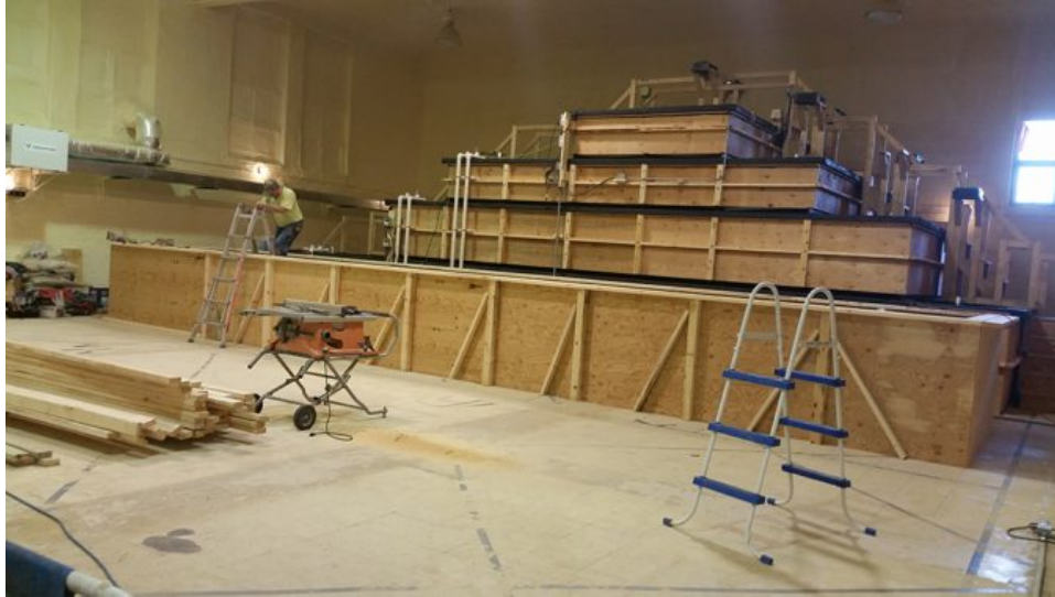
The indoor shrimp farm built by Sherlock Shrimp is using a tiered tank system in which the shrimp, as they get larger, move from the smaller tanks up top to the larger tanks below. Courtesy photo.
