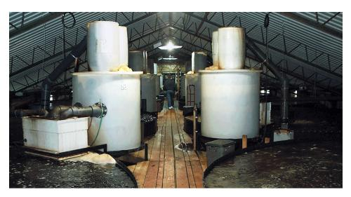
Eastern Tilapia's recirculation system features growout tanks with packed columns, biofilters, and low-head oxygenators.
