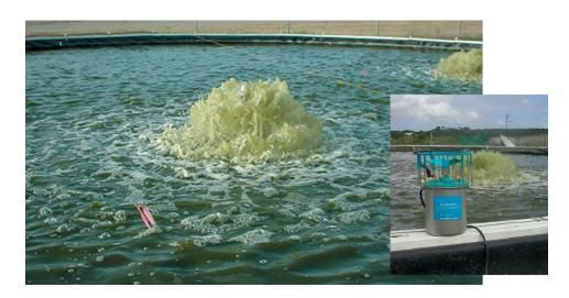
Vertical pump aerators provide good localized oxygen transfer.
