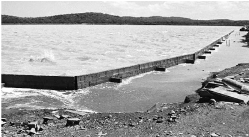
High rates of erosion from wave action greatly increase inorganic suspended solids loads in ponds.
