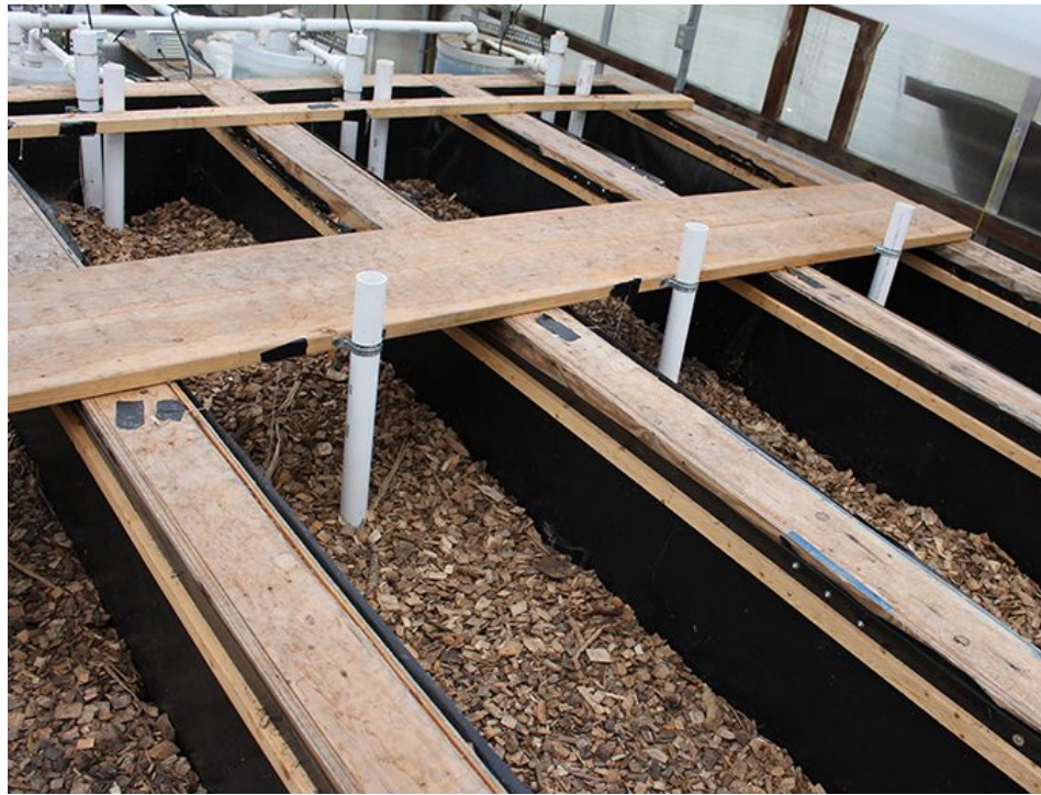
Four experimental pilot-scale denitrification woodchip bioreactors, located at The Freshwater Institute in Shepherdstown, West Va., USA. The bioreactors here are sized to be 1/10 scale of a field reactor.
