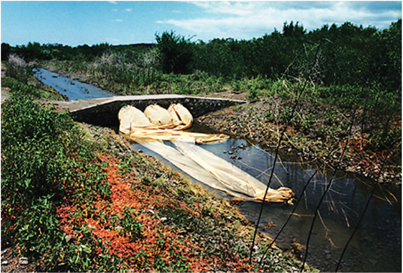
Incoming water flowed through a series of filters to eliminate hosts that could harbor shrimp viruses. Photo by Russ Allen, Michigan Sea Grant.
